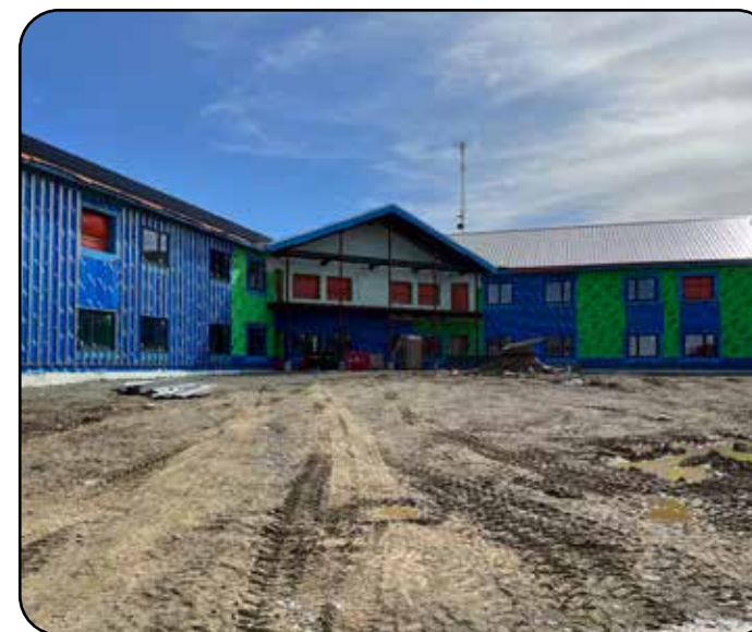
Villa Acadienne new Long Term Care facility building under way!
