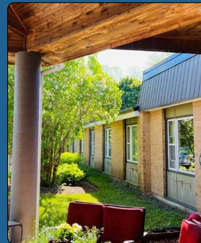
A Society favorite was the design and installation of the unique front entrance wooden awning. The beautiful awning gave a shaded area for residents to sit and enjoy the spring and summer in all its glory.
